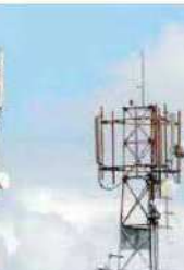
Mobile tower structure.
