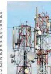
Mobile tower structure.
